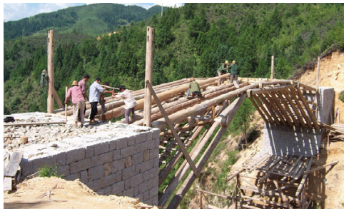
Fig. 6.5.4. Zheng Daoju, Construction of traditional beam-woven structure
