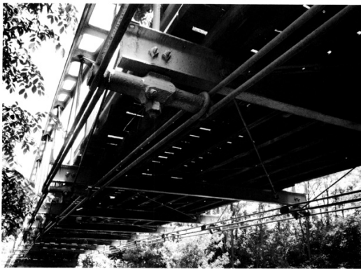
Fig. 1.5. Detail of the combined use of cast and wrought iron in the Whipple bowstring arch at Claverick, New York.
